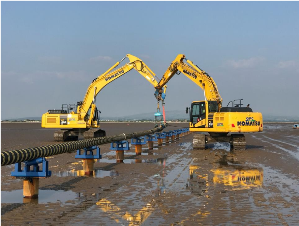
Plate 4.3 Example of cable being pulled ashore by winch supported by excavators
